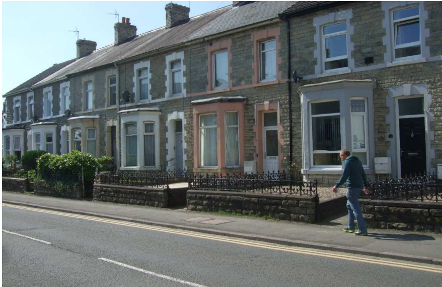
Fig 2: Streetscene view of property
